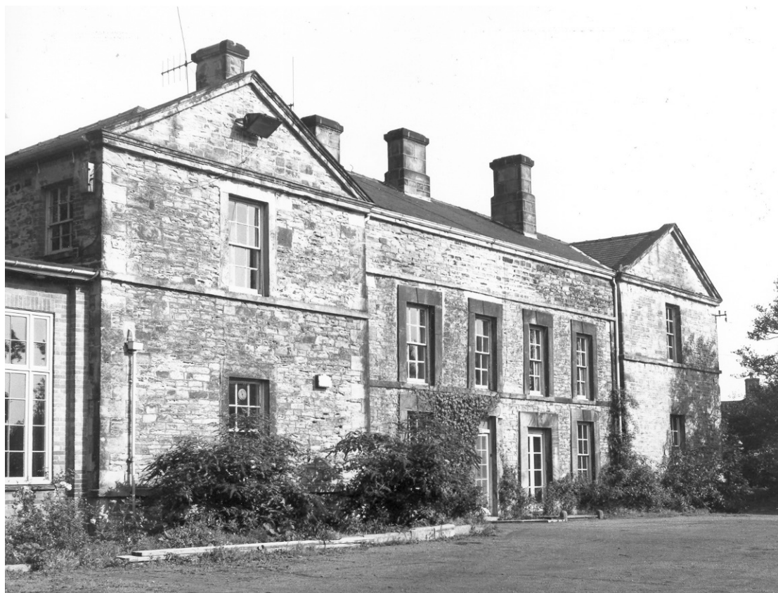
Figure 398: Former Rectory, Handsworth - built in the late 17 th or early 18 th century, but containing part of a cruck timber.
